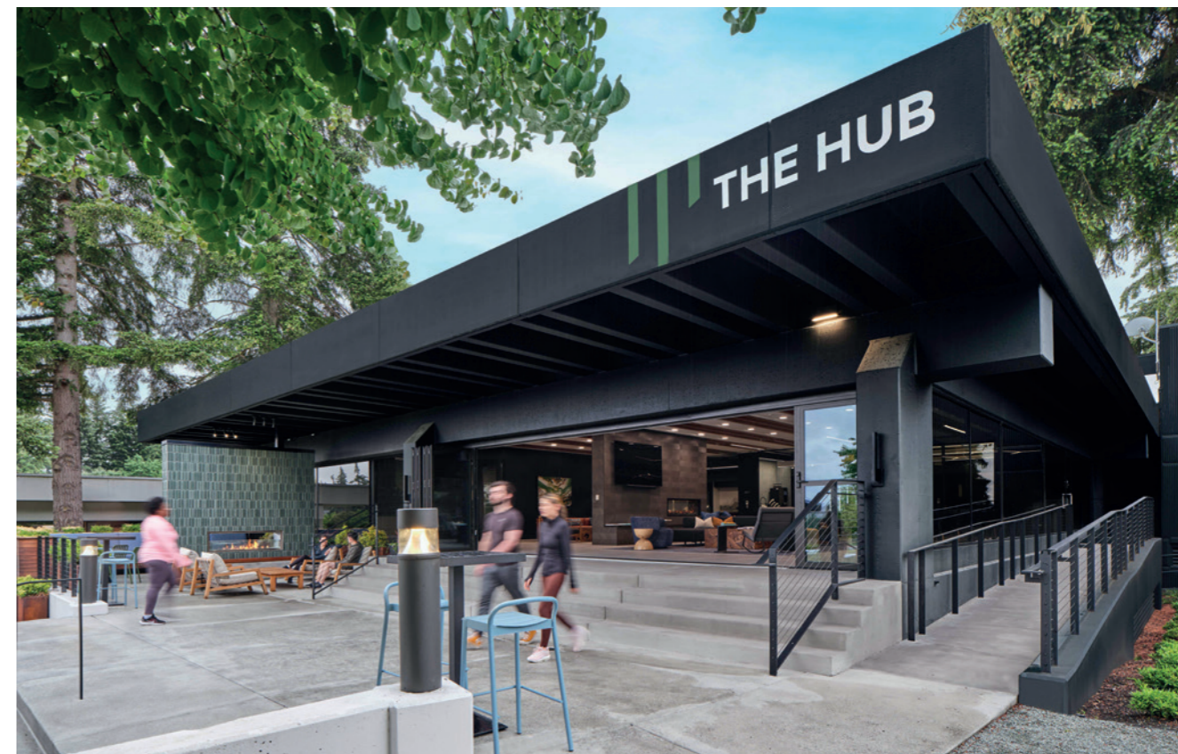
The Hub at Bellevue Technology Center, Eastside Bellevue, is a freestanding amenity building within the campus.
