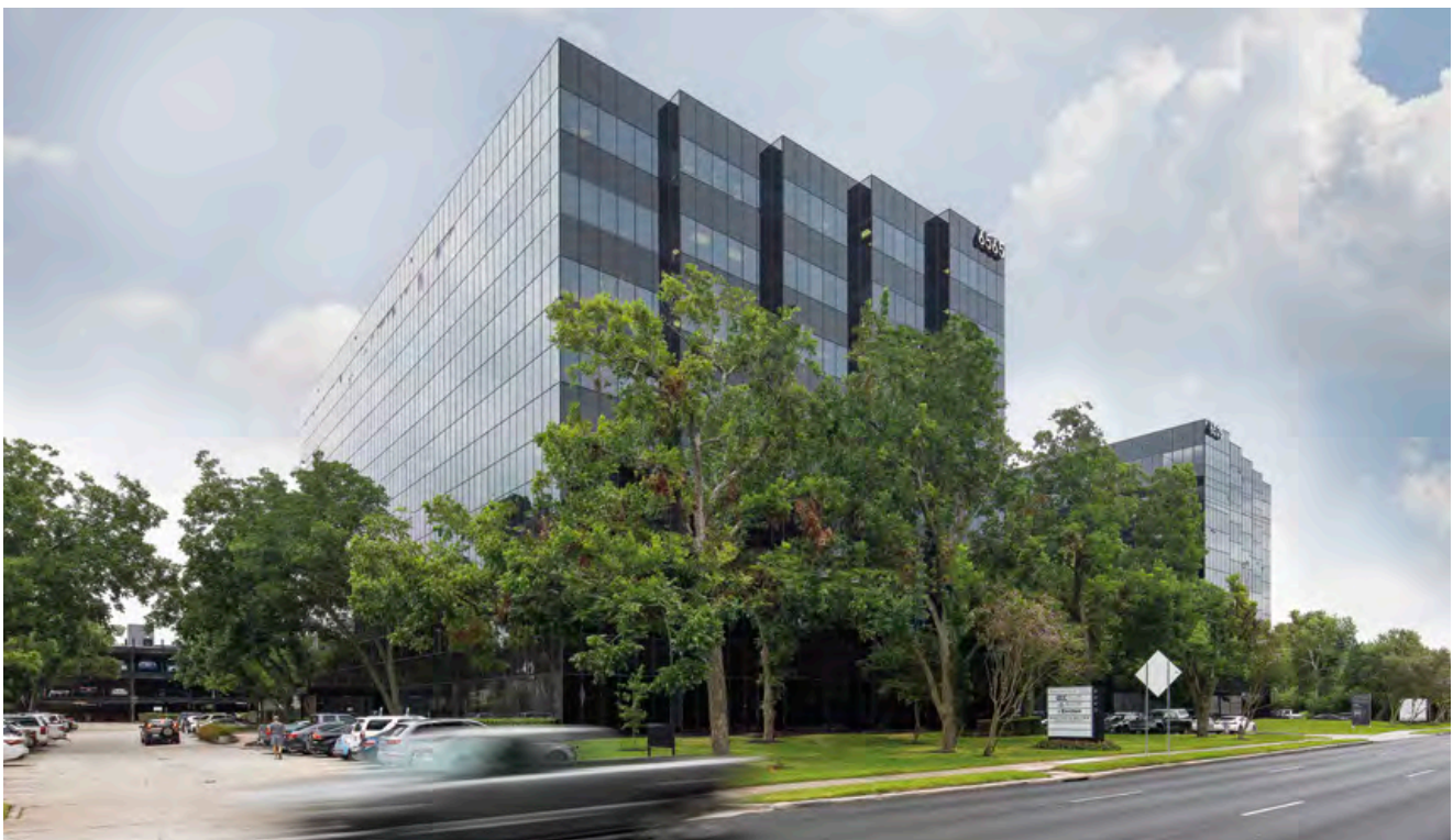
As at 31 December 2020, KORE has a balanced portfolio of 13 office buildings and business campuses in the US, including Bellaire Park (pictured).
