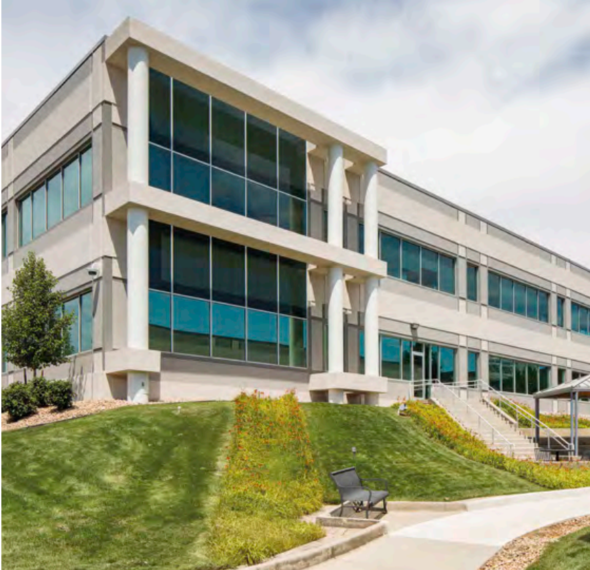
As an affirmation of excellence in sustainable performance, Westmoor Center (pictured) is a recipient of the US Environmental Protection Agency's ENERGY STAR® label.
