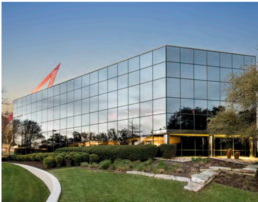
The Manager is committed to active stakeholder engagement, including with tenants at its properties. Pictured is Westtech 360 located in Austin, Texas.
