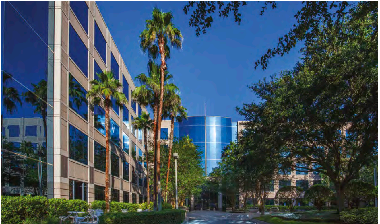
Several energy and water management initiatives were implemented at Maitland Promenade I and II (pictured) in 2020, including the progressive upgrade to LED lightings and installation of low-flow, auto sensor faucets in the buildings.
