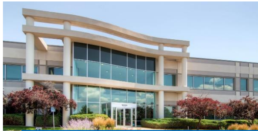
Westmoor Center, Denver
